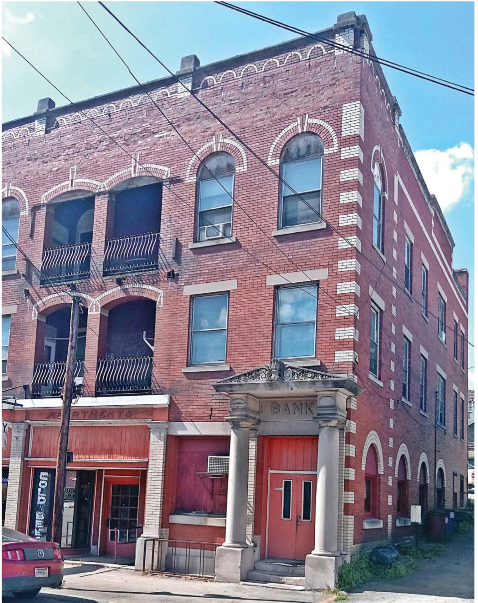
The Farmers and Merchants National Bank of Rockwood was across the street from the First National Bank. It occupied an older block, as it was the successor to the Rockwood Savings Bank. Here is how the building appears in Rockwood today.
