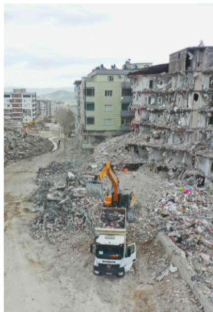
A work in progress
